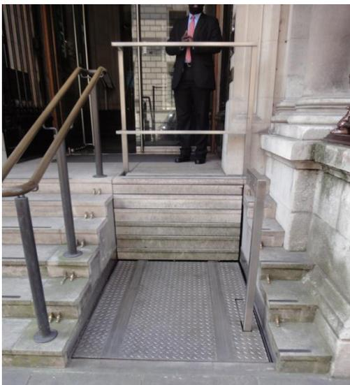
This picture shows the steps when they have receded and the wheelchair lift is in the position to transport someone into the front door of the building.
